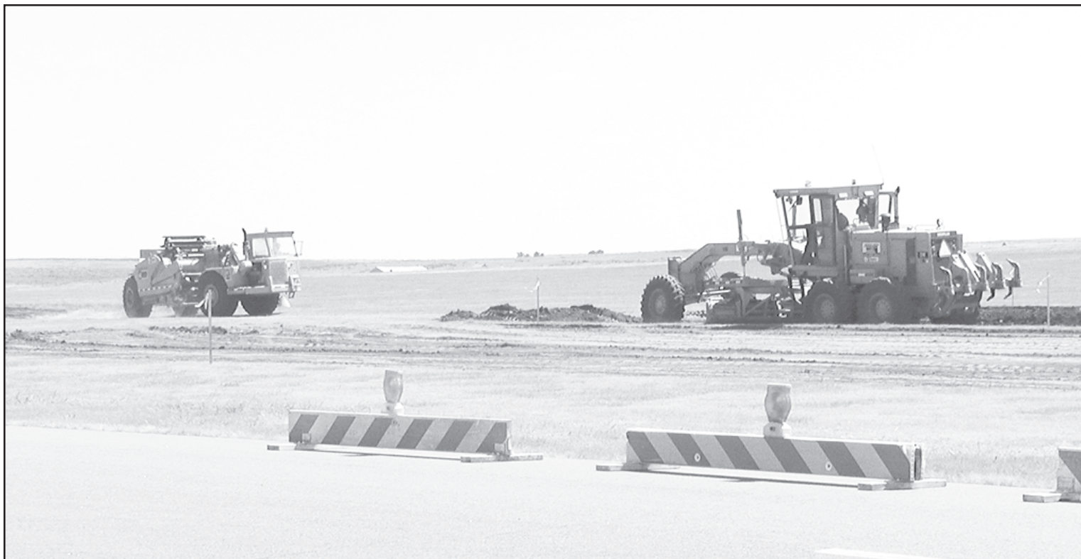
TUESDAY was the start of the dirt work for the construction of the apron which will allow for more parking area for planes.
