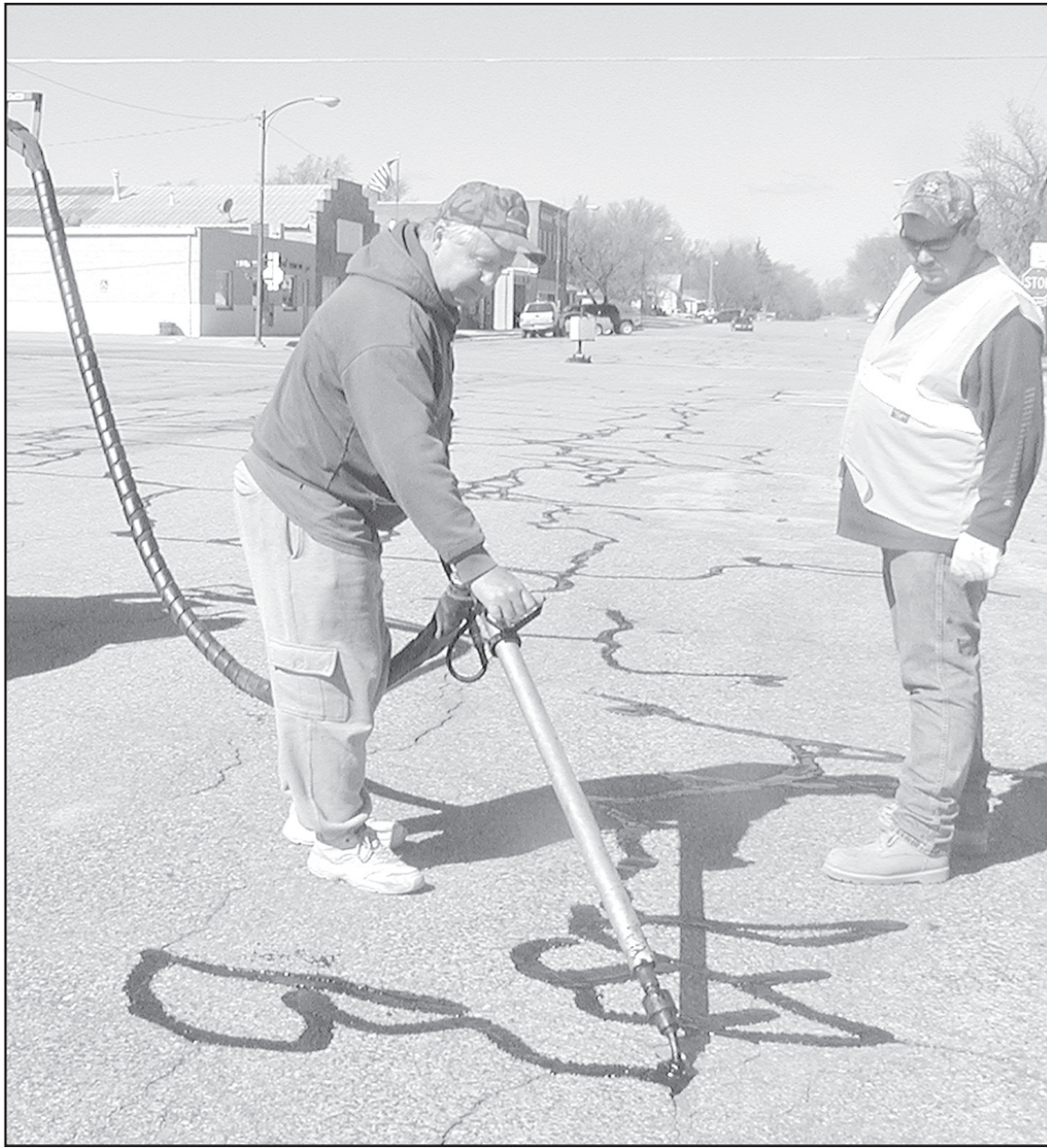
CREWMEN FROM KAUFFMANS'S SEALING COMPANY, have begun the work of sealing street cracks in Bird City.
