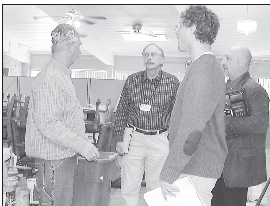
INSPECTION OF REMODELING was done Thursday. Pictured, l to r, are Don Post, site supervisor, Altman Charter, Jeff Paulsen, Village administrator; Eddie Stechsultz, project engineer, Altman Charter, and Leonard Kemnitz, engineer, Good Samaritan Society.
