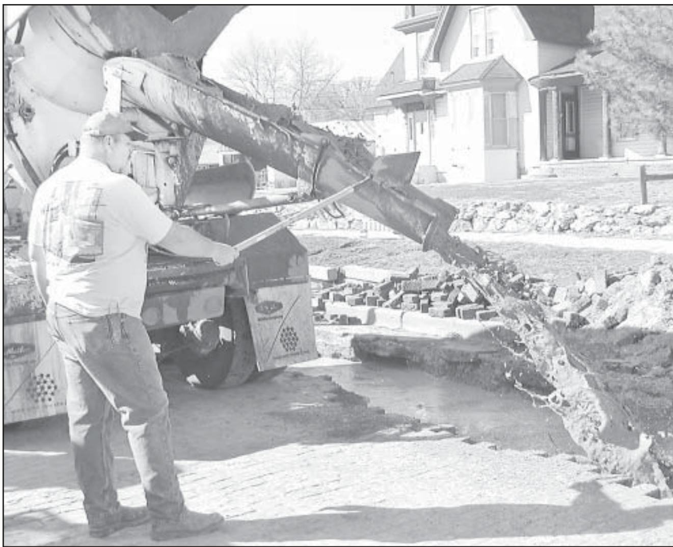
A Norton city crew worked to repair a break in a water line, which caused the city's water to be turned off for a couple of hours on Tuesday. Once the break was repaired the hole had to be filled in. Steve Reedy (above) steadied the concrete as it came out of the mixer and then shoveled it (below) while Mike Cliff and Ed Lively put up barricades. — Telegram photos by Veronica Monier
