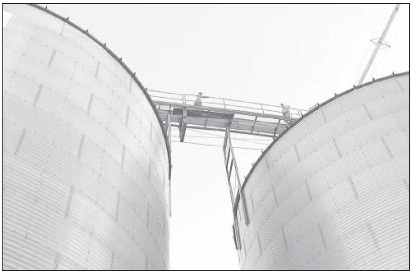
Nathan Donahey, elevator operator at Reager for the Norton Co-op, and Don Jones, employee, went top-side Wednesday evening to tighten the drag conveyor on top of the bins.
