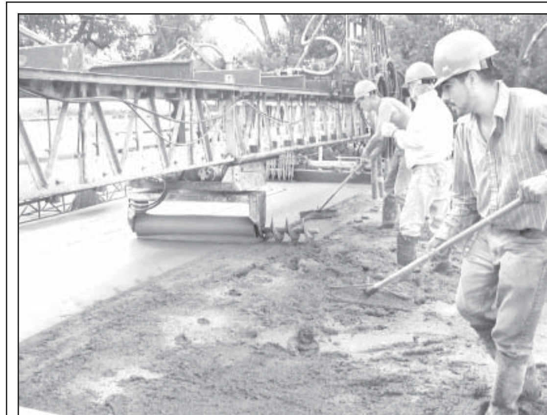
The work crew for Reece Construction Company, Scandia, poured concrete Wednesday morning for the south side of the bridge west of Norton. A power screed smoothed and spread the mixture before a workman with a bullfloat put the finishing touches on it. — Telegram photos by Carolyn Plotts
