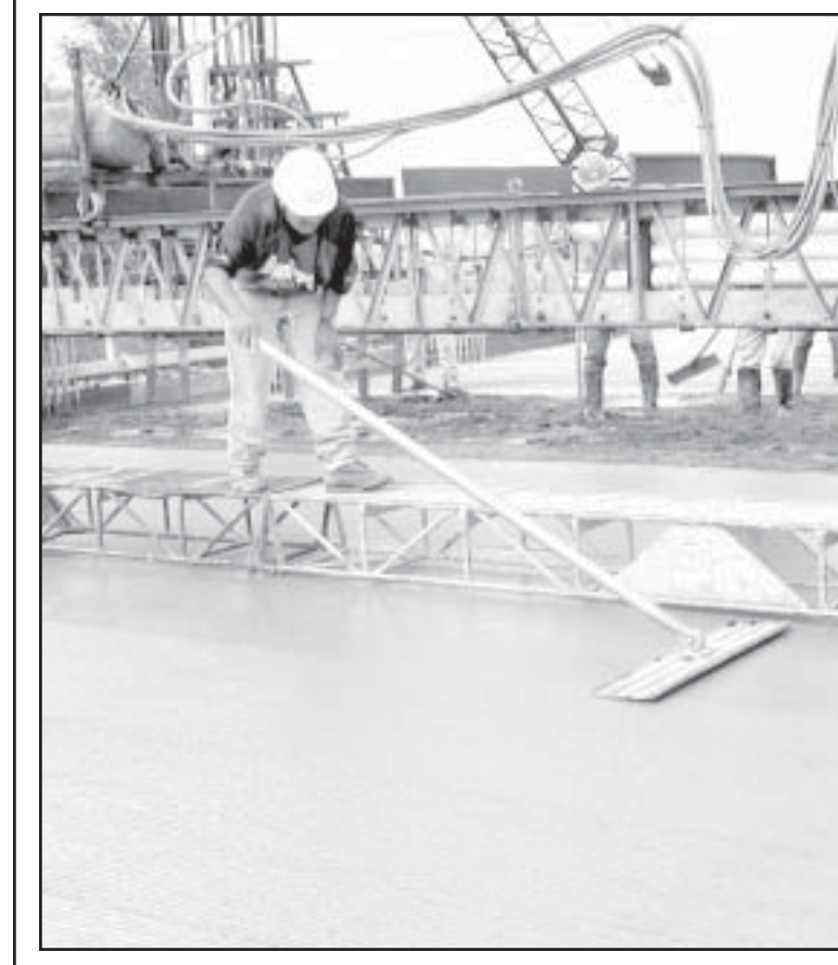
The work crew for Reece Construction Company, Scandia, poured concrete Wednesday morning for the south side of the bridge west of Norton. A power screed smoothed and spread the mixture before a workman with a bullfloat put the finishing touches on it. — Telegram photos by Carolyn Plotts
