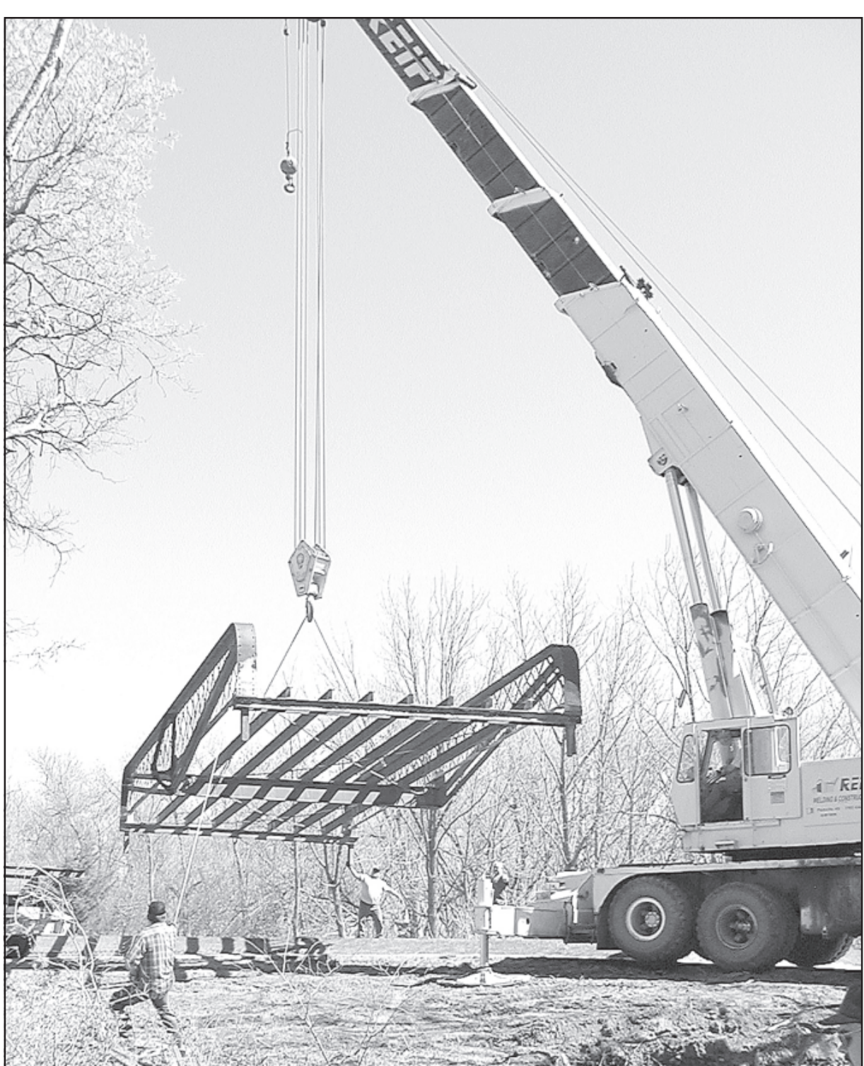
Norton County Bridge OS-75 was moved last Thursday because of its historical significance. The bridge's frame was transported via county roads to the Prairie Dog Golf Course, where it was lifted into place (above) by Reif Construction. Nelson Brothers Construction (below) helped to get the bridge set in place so it could be reassembled.
