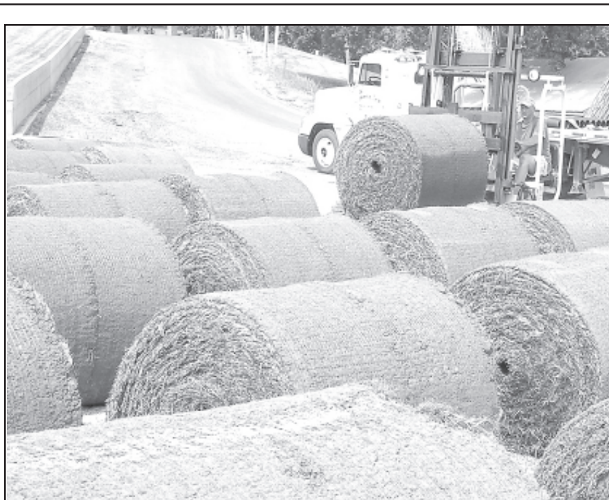
The Norton School District is "overhauling" the football field. On Thursday, 30,000 square feet of the 60,000 square feet of sod arrived in Norton. Each roll of sod is 4 feet wide and 120 feet long.
