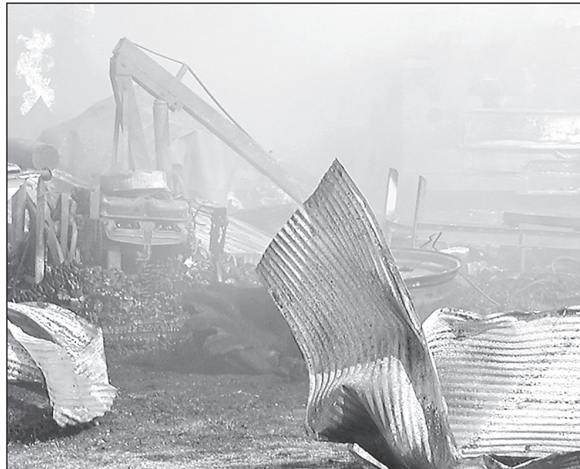
A fire completely destroyed what was once Don and Marilyn Lowry's shop garage Friday afternoon.
