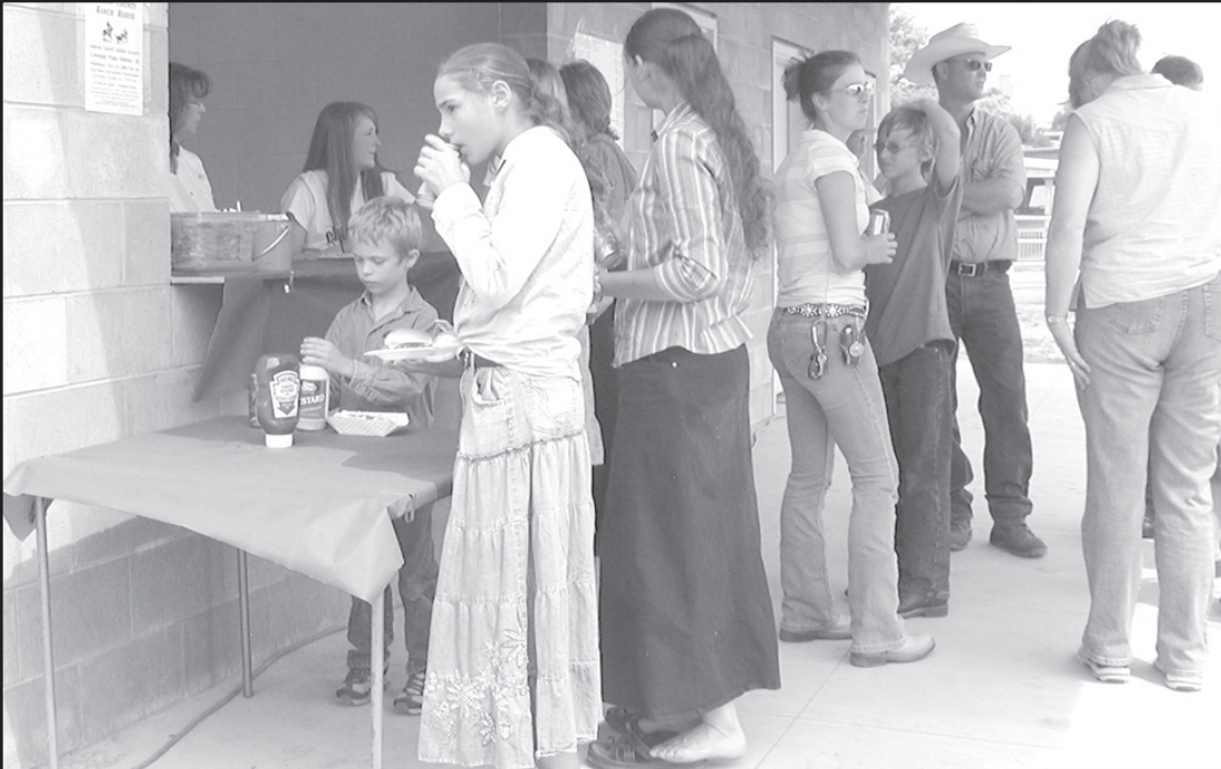
The new concession stand at the Equine Center at Elmwood Park proved its worth last Tuesday during the District 4-H Horse Show. Members of the Norton County Horse Council operated the stand serving food out of the almost-completed facility. Appliances are still to be installed and the showers need to be finished.
