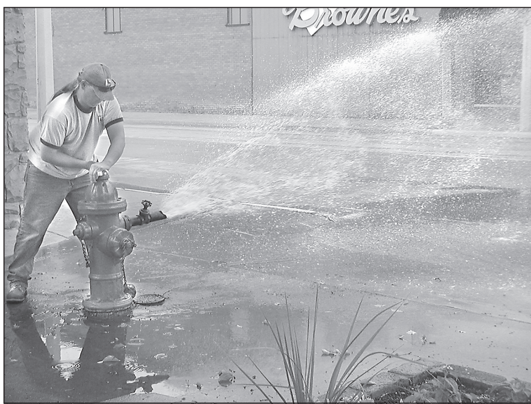
Jason Dial, city employee, flushed fire hydrants around town, and on Tuesday turned it loose at the intersection of Main and State in the downtown area.
