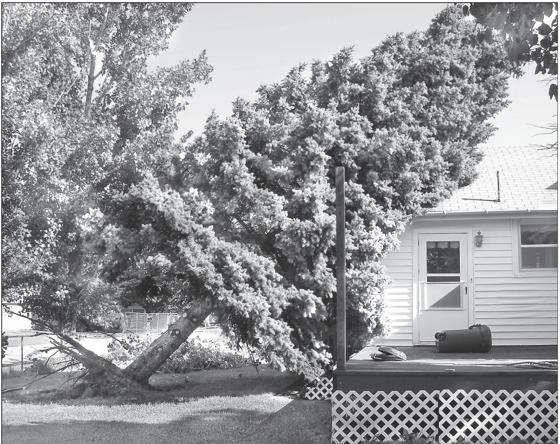
It almost looks like this giant Christmas tree was trying to get into the house, but the wind-driven storm Saturday night beat it to the punch, ripping it out of the ground and shoving it onto part of the roof of the home at 613 W. North Street. The wooden fence at the Dan Pfannenstiel
