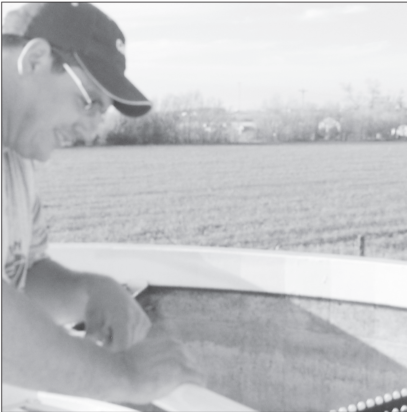
Chris Frack, water plant supervisor, demonstrated the water clarifier at the water plant. All water comes into the tank which removes mud and other debris before the water is purified further. The tank, which is usually full, is empty due to the problems with the clarifier. The issue was discussed at Wednesday's city council meeting.
