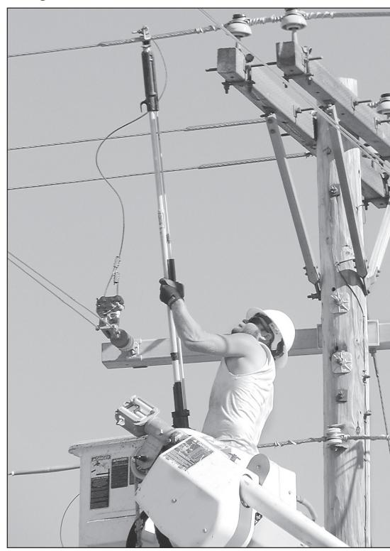
Working high in the air, Spencer Schenk of Ainsworth, Neb., used multiple safety devices to work on a "hot" power line on the Upper Dam Road just off U.S. 36 last week. The work is part of the Federal Emergency Management Agency's effort to replace power lines in the area. The line is owned by Prairie Land Electric.
