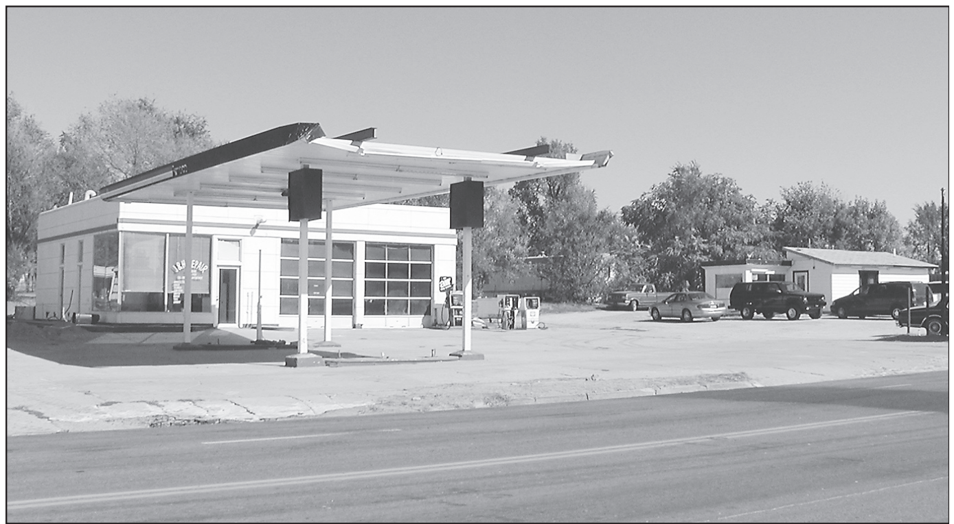
The former filling station and Beacon Cafe buildings will be demolished to build a new hotel.
