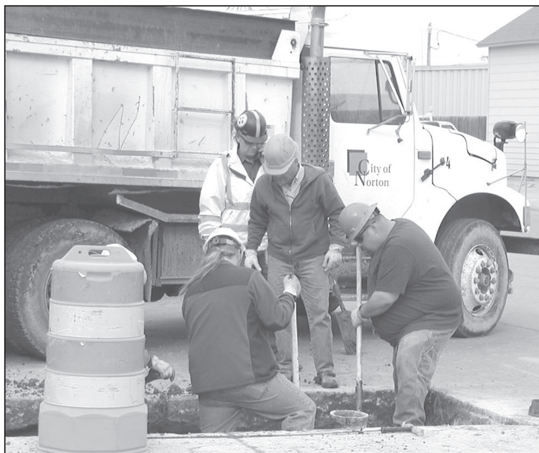
The employees of the City of Norton have had their share of fixing broken waterlines since winter started and even before that. Pictured here is a crew mending a 12 inch water main that has had a small water leak at a joint for some time. The work being done was located at the corner of State and Lincoln in Norton. - Telegram photo by Dana Paxton
