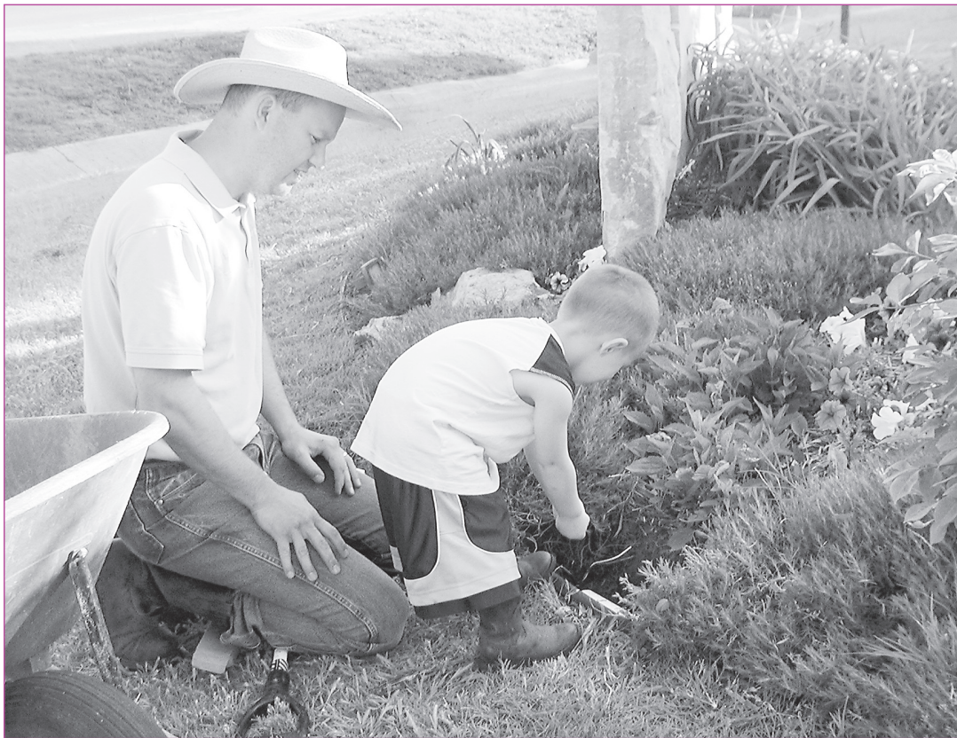
Aaron and son Gideon White do some repairs on the flag lighting in front of the Norton Animal Health Center. Beautiful flowers and a lit flag on the Center's corner welcome everyone to the west edge of Norton. —Telegram photo by Dana Paxton
