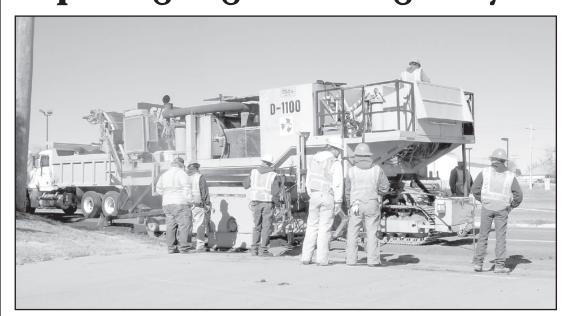
Kansas Department of Transportation crews were hard at work Tuesday afternoon to repave a section of Highway 36 through Norton. The work included milling off a layer of the asphalt and installing an overlay on a section of roadway from West Street in town, extending east to the city limits. -Telegram photo by Carlleen Bell
