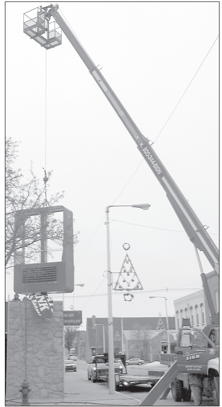
Workers from Commercial Sign Company in Colby braved brutal rain and cold Monday to take down a large sign at First State Bank in Norton. The signs are being removed from the bank building to be cleaned and refurbished. The sign will get a new canvas and lettering, then be re-installed at the bank at a later date. The sign had to be lifted off the building by a crane on State Street.
