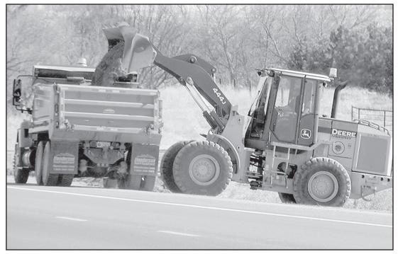
Kansas Department of Transportation crews were hard at work Thursday afternoon on Highway 36 a few miles west of Norton. The crews were working to build up the shoulders of the road and moving dirt around to improve drainage around some bridges on the highway. Though winter weather is predicted for today and tomorrow, the weather was perfect for working outside Thursday afternoon.
