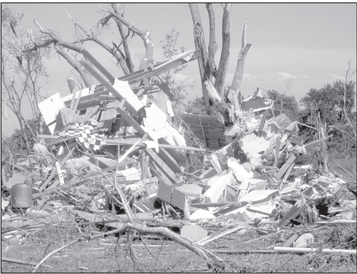
An EF-3 tornado swept through Norton County on June 20, 2011, leaving widespread destruction. This home just northeast of Alma was blown from its foundation and mangled beyond recognition during the storm. No one in the home was injured.
