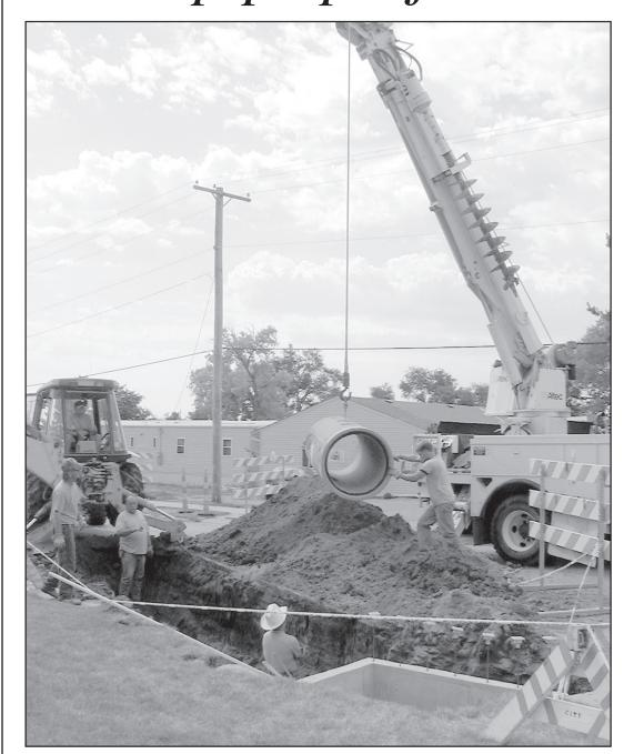
On June 9, the Norton City crew started a drainage job near the corner of West Crane and Nixon. A new drain pipe was laid along the side of the street as well as under it to divert water around Holly's Clubhouse. Workers are seen here lowering the new drain pipe into position.
