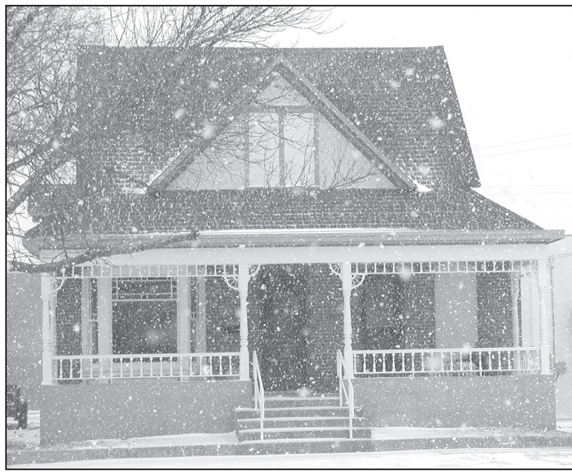
The Lyons house has been under restoration for over a year now and it has been a leading story throughout the year. The home has withstood many winters in its lifetime and now it looks as if it has a second chance at life and will see many more winters.
