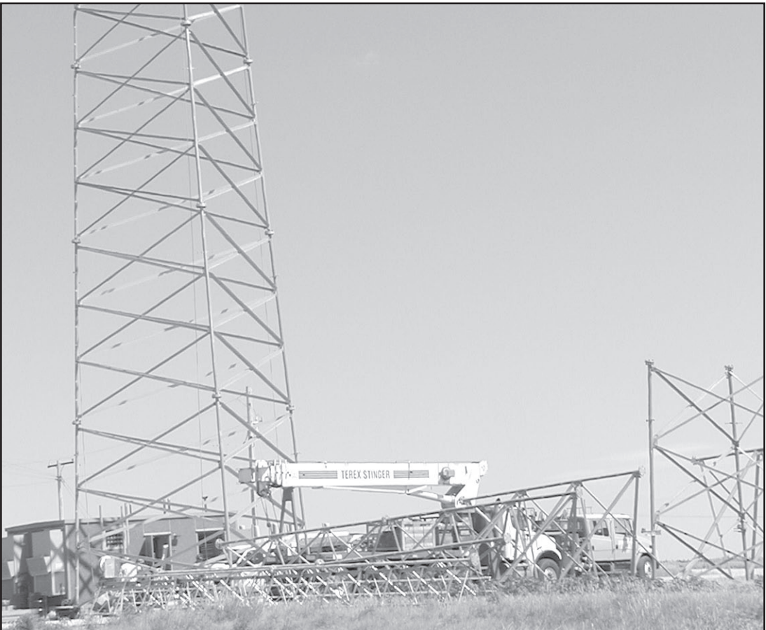
A 280-foot cell tower is being erected at the Norton-Decatur county line across U.S. 36 from Norcatour. The tower is being built by Hayden Tower Service out of Topeka and will take another week to week and a half to complete. The tower is for Verizon and will carry a 4G system.
