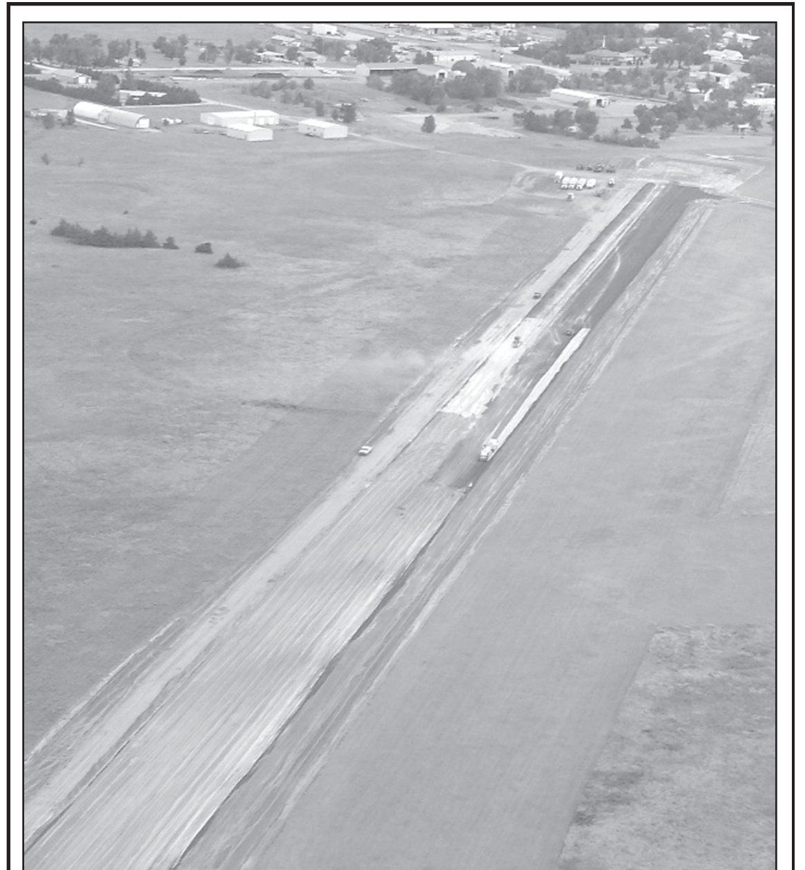
AIRPORT RUNWAY RENOVATIONS are moving right along. Robert Grace, who took the aerial photo said the contractors have removed all the asphalt, piled it up, ground it up and completed the dirt work. They are now reincorporating that ground up asphalt into the dirt as a base for the concrete. The runway is expected to be completed by Oct. 17.
