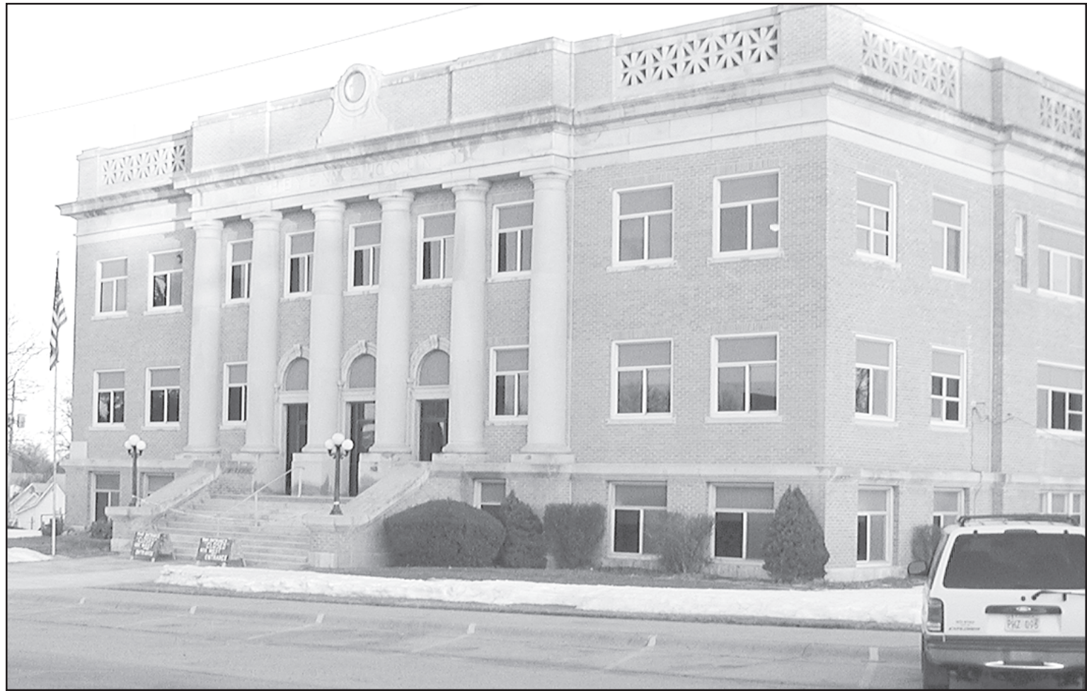
OVER 80 YEARS OLD , the Cheyenne County Courthouse is a well-kept, beautiful structure. All that is needed is new steps.
