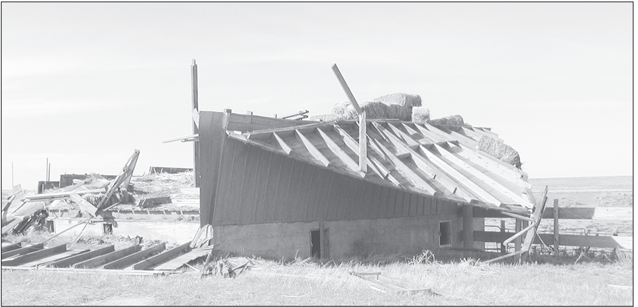
The sides of Bud Mears' barn were torn off and laid on their sides. Notice the hay bales in the loft that the tornado left behind Photo by Melinda Basnett
