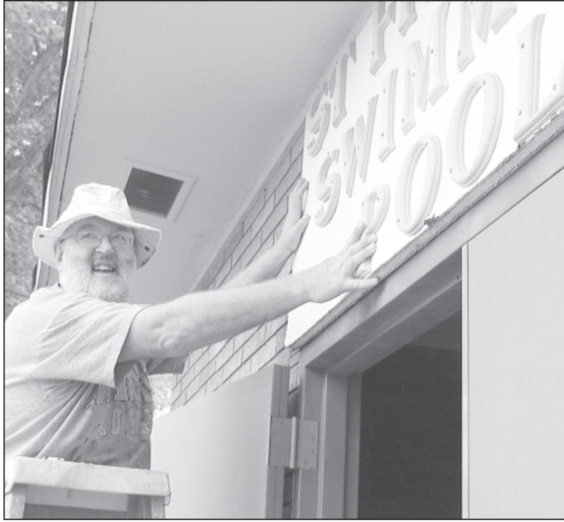
BRUCE SWIHART takes down the old sign that needs repairs at the swimming pool.
