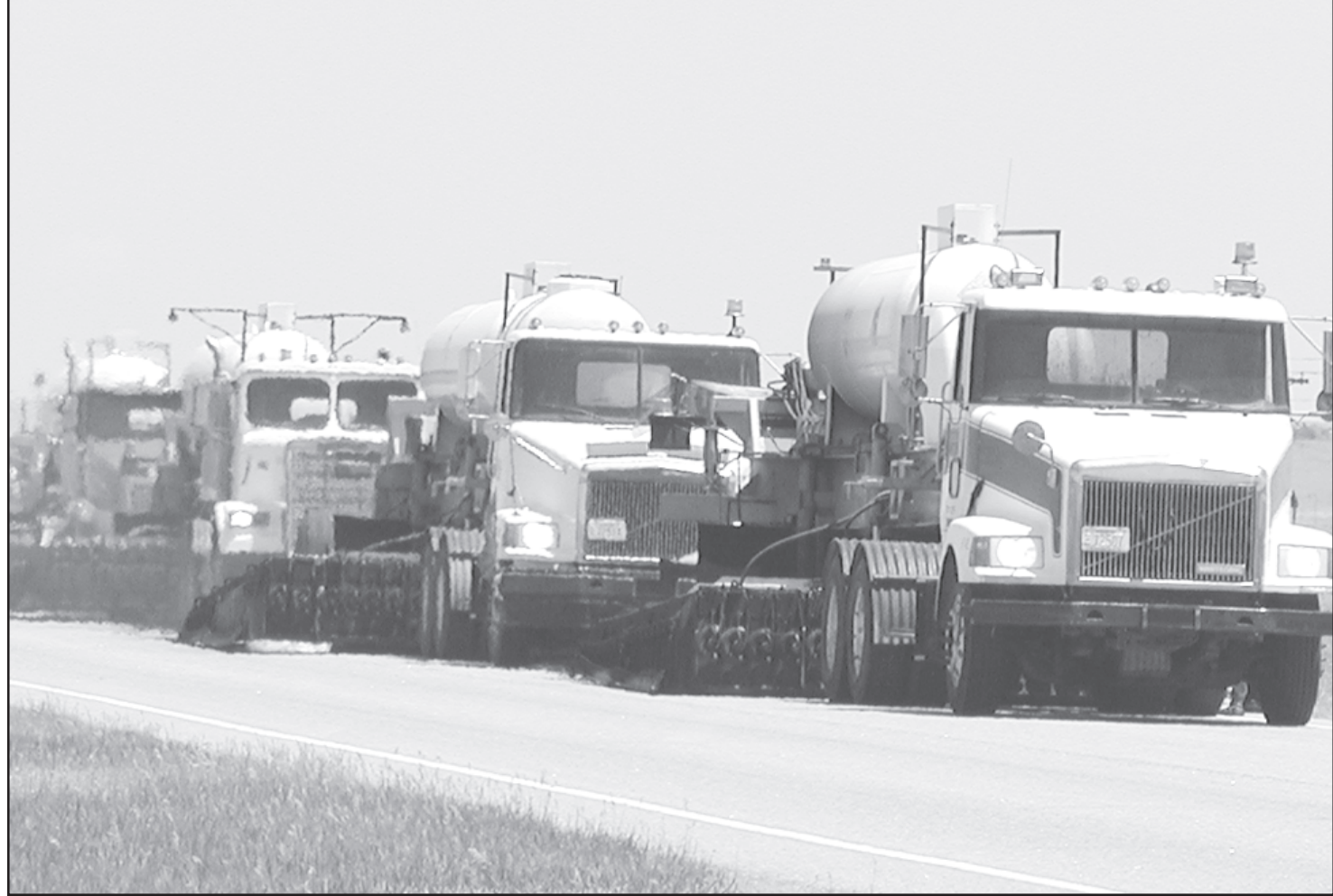
ROAD CONSTRUCTION is well underway west of St. Francis as the crew works their way to the Colorado line. The recent rains have slowed the progress somewhat. Herald staff photo by Karen Krien
