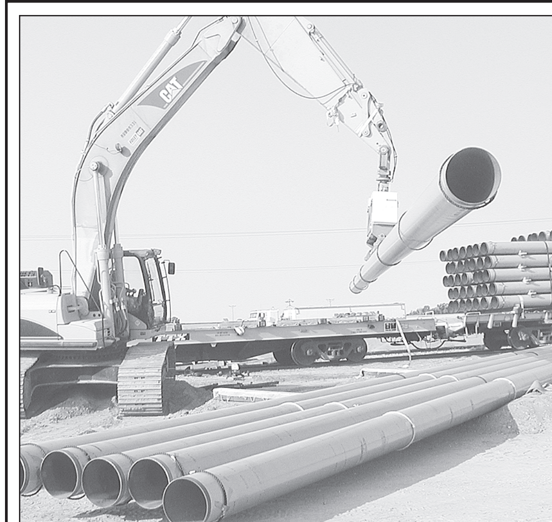
PILES OF PIPE — 16-inch pipe for a natural gas line are unloaded from rail platforms in Bird City. About 40 platform cars of pipe were also delivered to McDonald.
