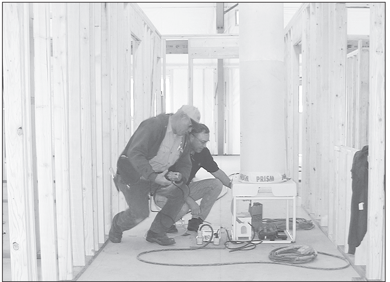
WALLS ARE GOING UP! Sam Miller and Kelly Frewen work inside the new emergency building. Walls were prefabricated off site and then brought to the new structure to be raised. Volunteers
