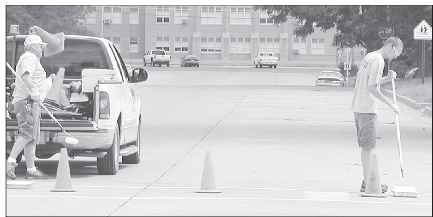
CITY WORKERS Glenn Schliep and Paul Larson repaint the cross walks around the school.
