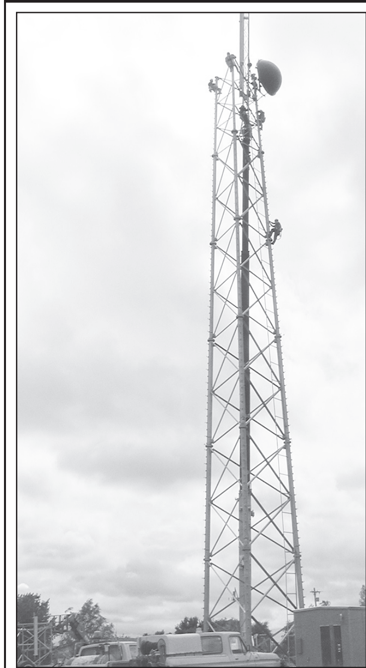
NEW VIAERO COMMUNICATION tower went up Friday. It is located south of the county shop, out of the city limits.
