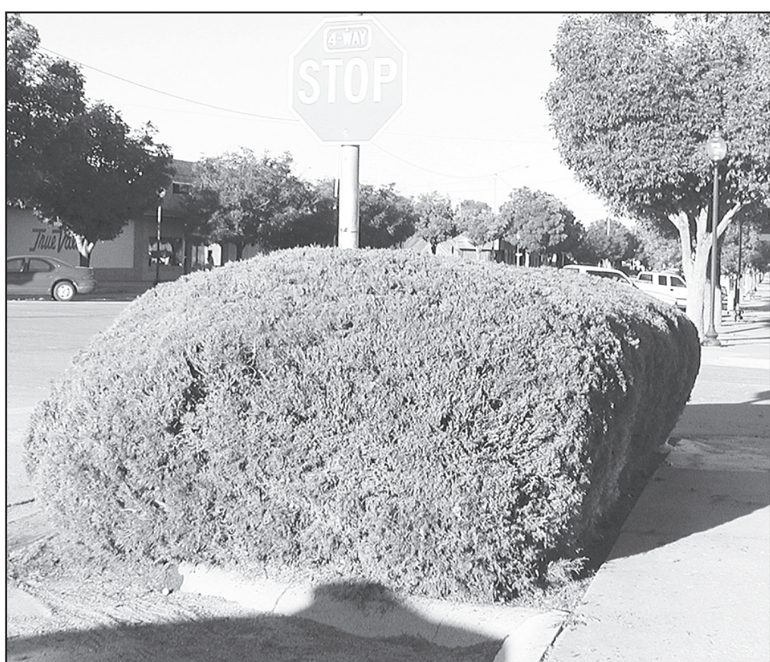
MYSTERY PICTURE — People were curious about why this bush made it in The Herald last week! Well, this is one of two bushes on either side of the courthouse. They are overgrown and hinder the view of traffic. The commissioners have tentatively agreed to have them removed and put in some different landscaping.
