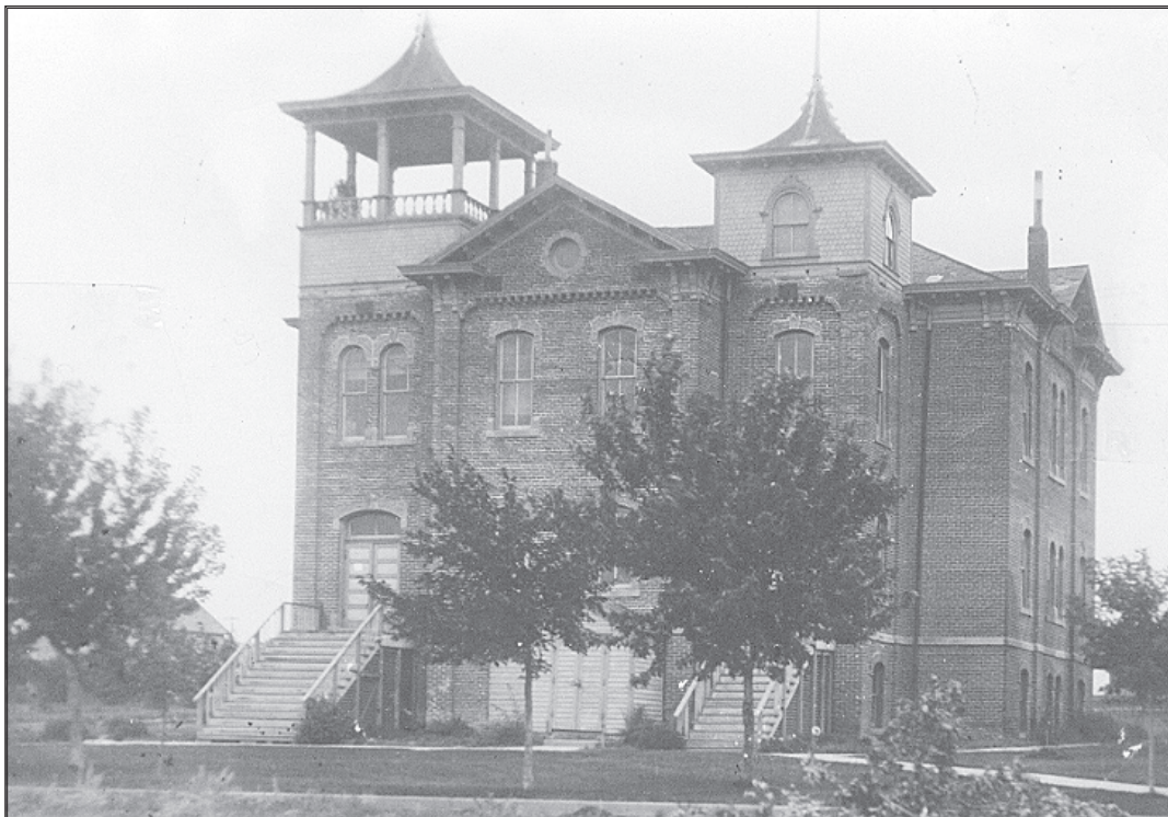
Early 1900 St. Francis school building. All grades 1-12 met here.
