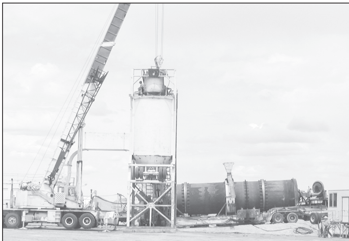
ASPHALT PLANT on K-27 is ready for work on Monday.
