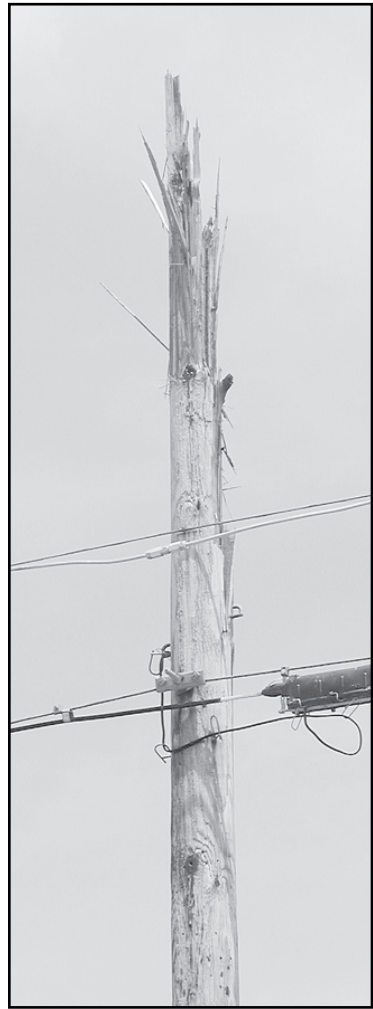
LIGHTNING STRUCK the phone pole near Fourth and Lorrwaine streets on Sunday evening.
