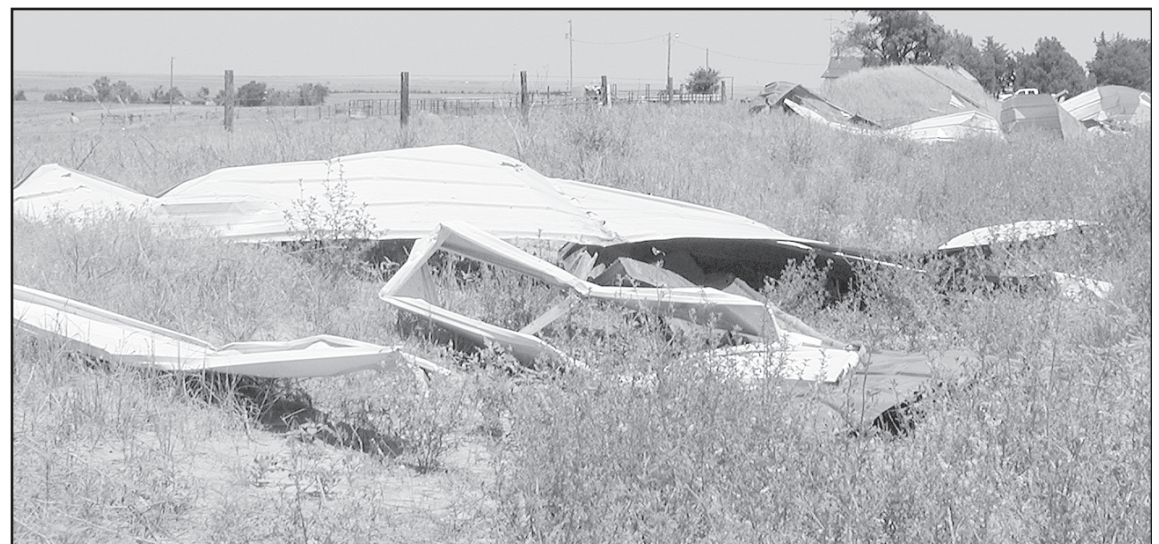
CARPORT MATERIAL was scattered along the ditch by the Brian Holzwarth home.
