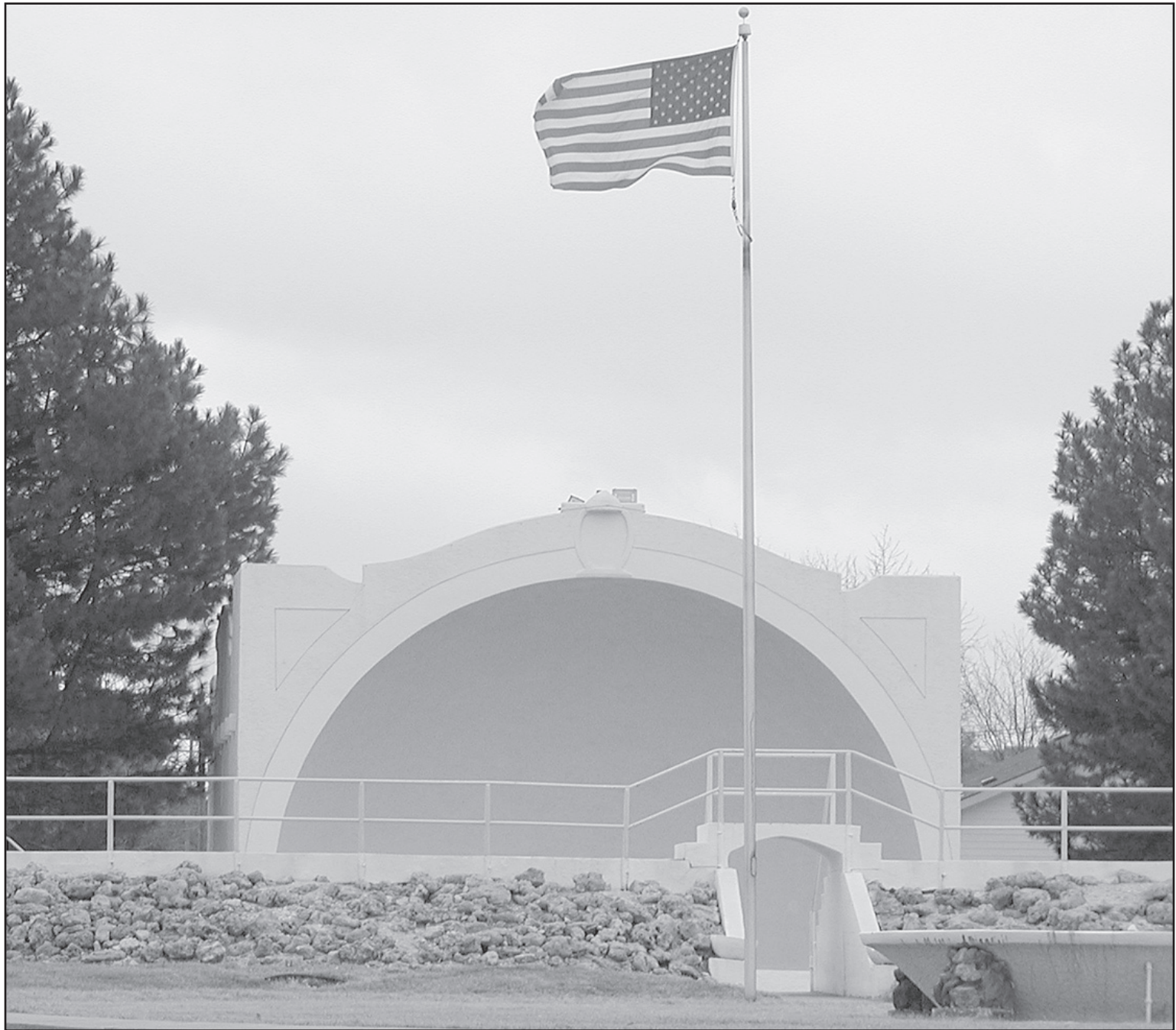
WORK WILL SOON BEGIN on the band shell in Sawhill Park. The band shell renovation was one of seven projects to receive the full money asked for from the Kansas His-
