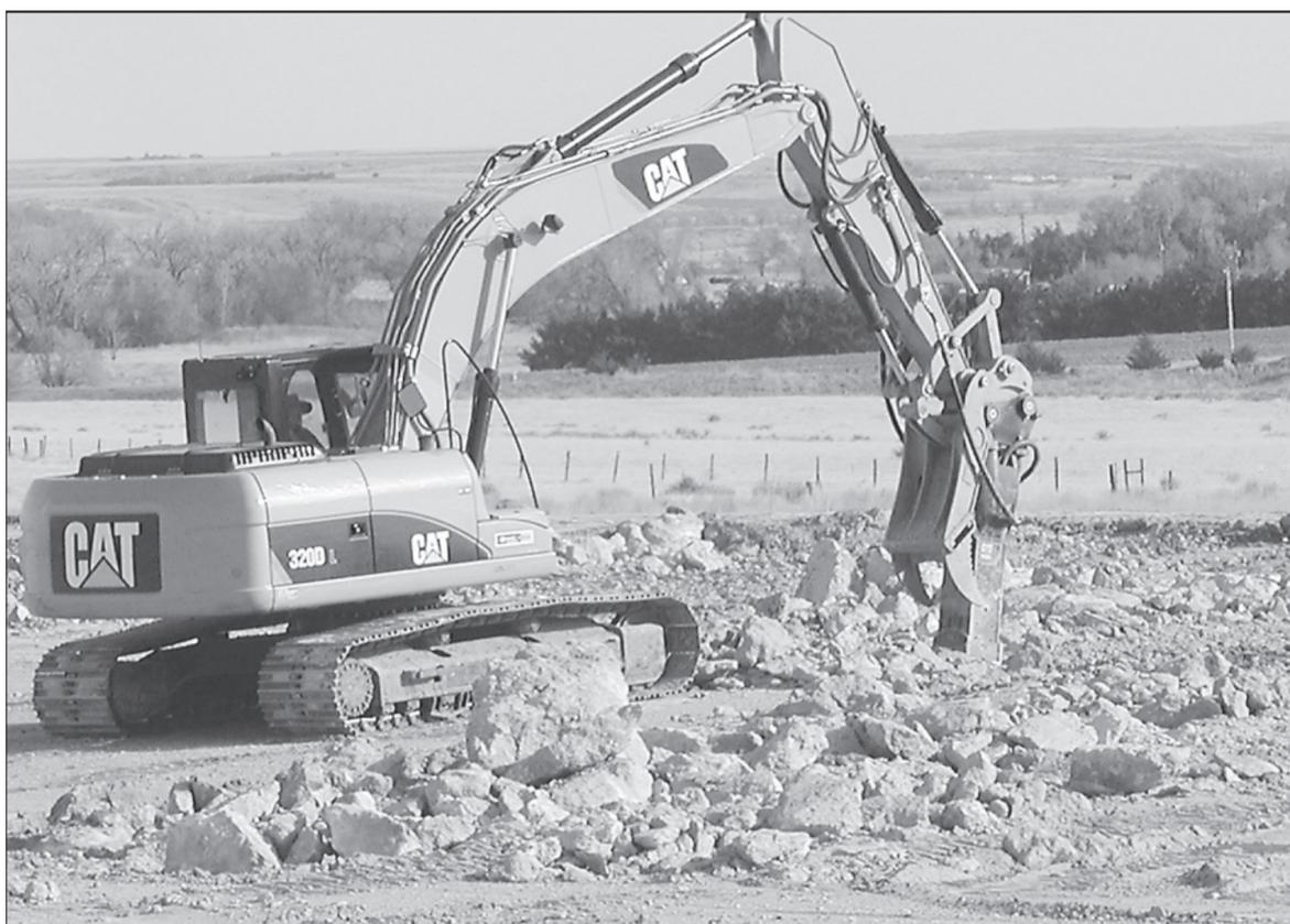
**SOLID ROCK** was found under a portion of the runway extension. This huge jack hammer was clearing away the rocks and loaders were hauling it off so the dirt work could be done.
