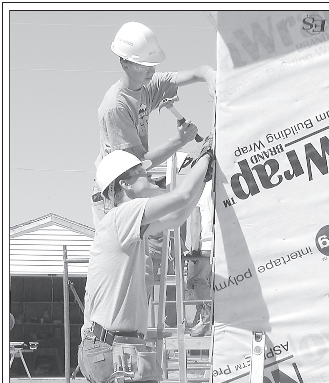
WORKING ON the wellness center were Joshua Keltz and Connor Hazuka on the ladder.
