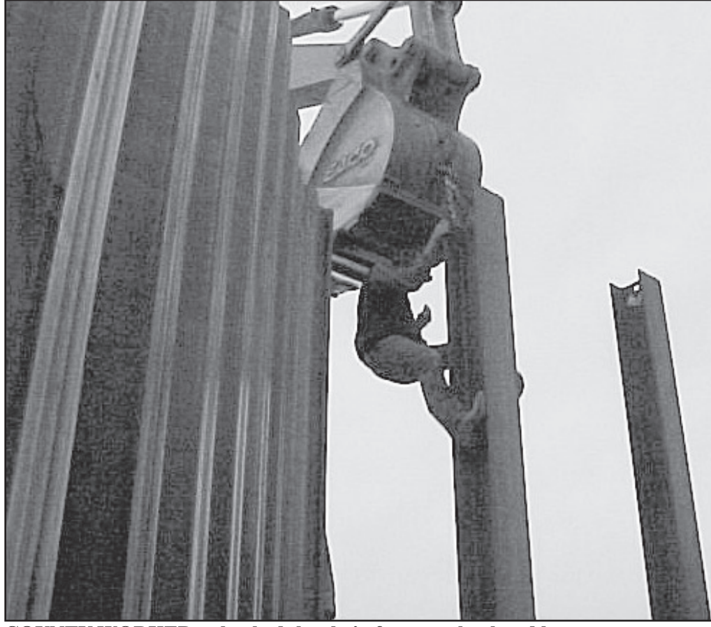
COUNTY WORKER unhooked the chain from newly placed beam.
