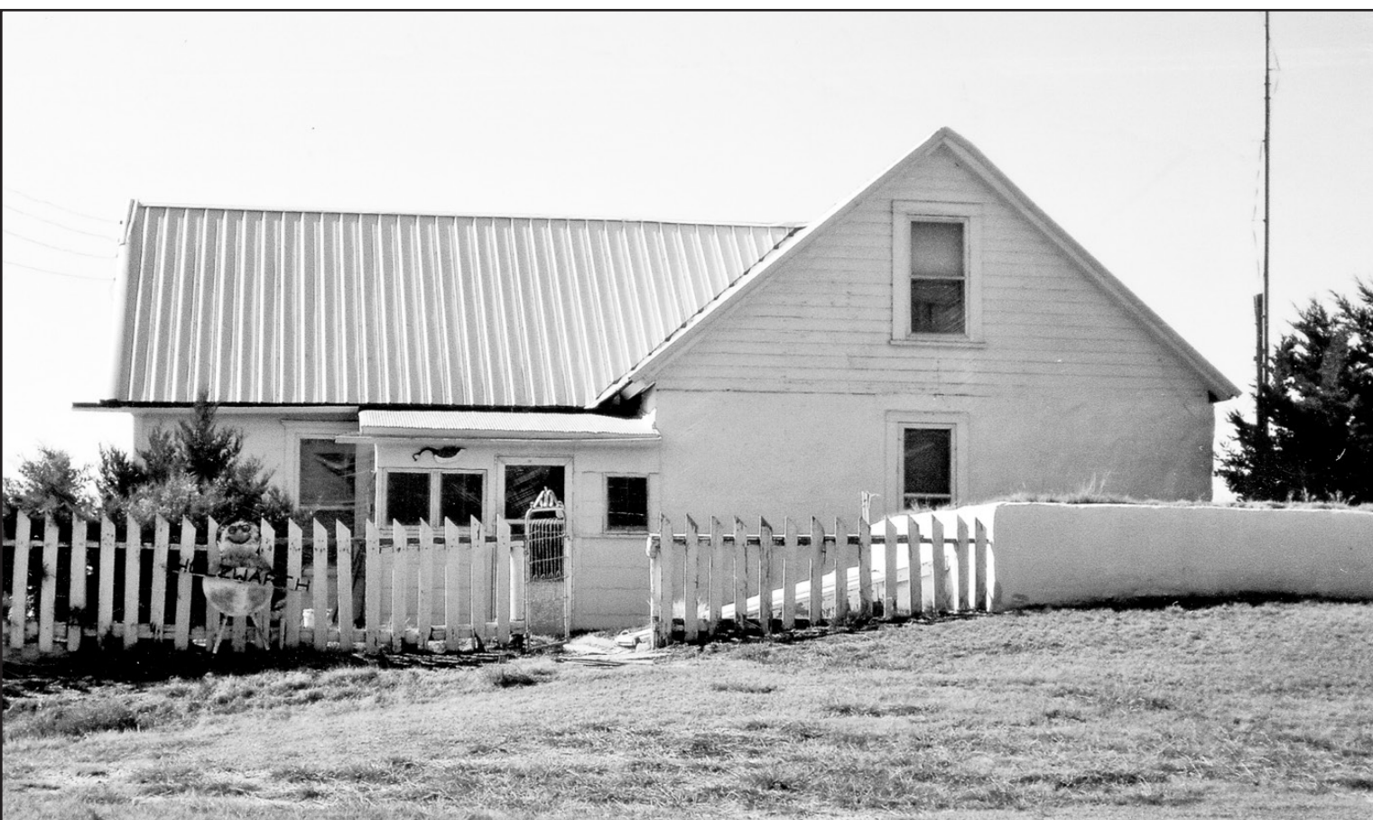
HOLZWARTH SOD HOUSE today. The sod is plastered over with cement, and additions have been made. However it is still lived in today.
