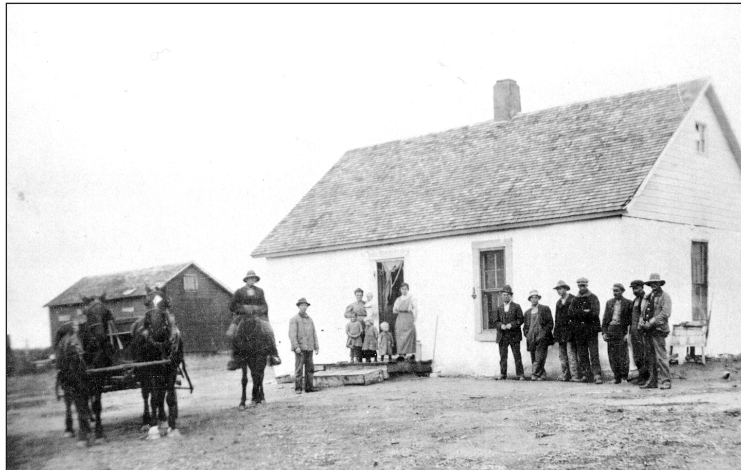
GEORGE HOLZWARTH FARM in 1915. George Holzwarth, with the help of his brother, John, built the house in 1907. George married Julia in 1908 and brought her from South Dakota to this home. The two rooms are made of sod and still lived in today. It has been added onto. The sod is preserved by the cement plastered over it.
