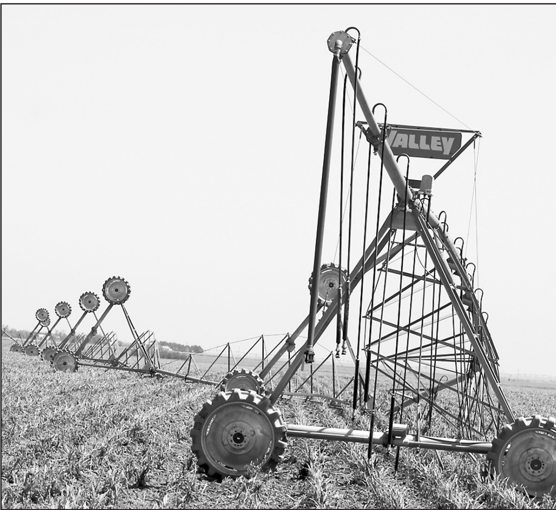
LYNN GLASCO'S sprinkler well was twisted and on the ground from the high winds that ripped through the area on Saturday evening. Reports of several center pivot systems being overturned have come in.
