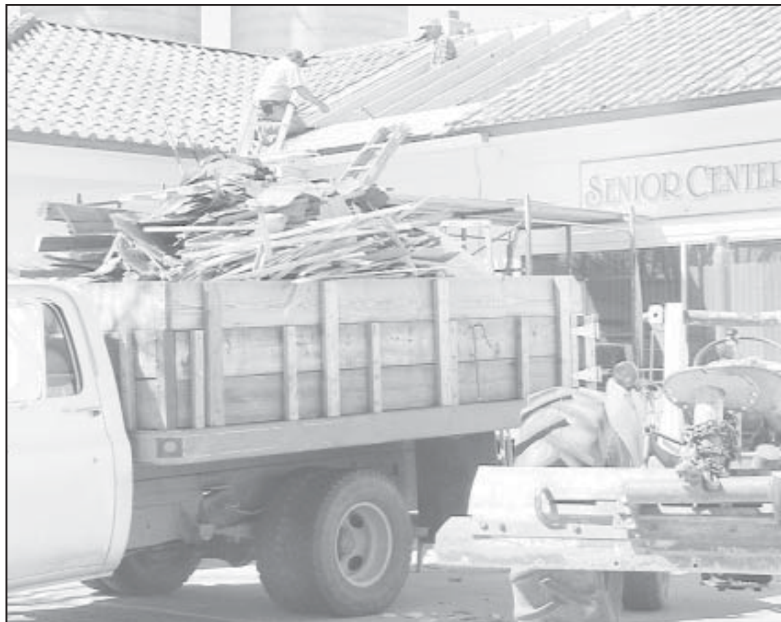
OLD TIN SHINGLES along with two dormers came off the senior center last week and Leon Merklin's crew put new shingles on. Doing the work on the roof were Brad Merklin, Chris Merklin and John Hankins. Herald staff photo by Karen Krien
