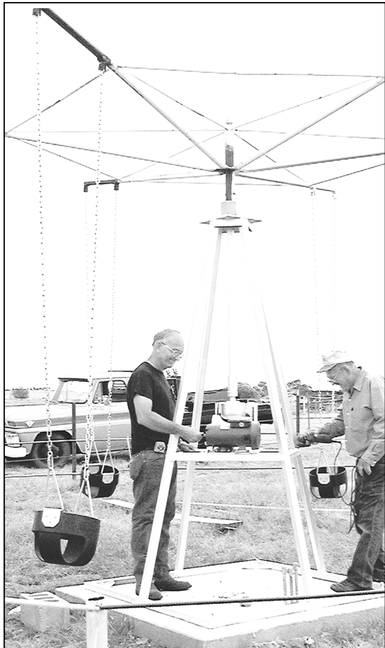
KID'S SWINGS was constructed by volunteers from leftover parts of the pony rides. Greg Walz, left, and Kenneth Knorr work on the motor. There are only a few more swings to install.
