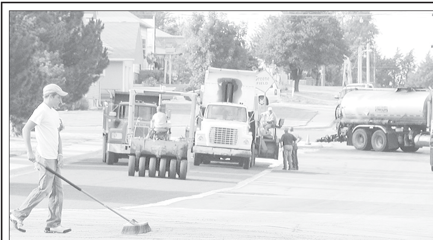
SEVERAL STREETS in St. Francis have been repaired the last week. The crew was busy sealing the street in front of the high school.
