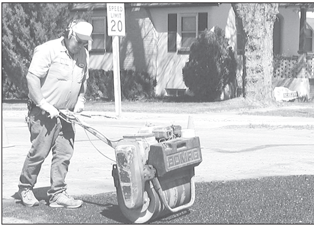
THE ASPHALT finally warmed up and Glenn Schliep, city crew, was patching an area of the street on River Street. Herald star photo by Karen Krien
