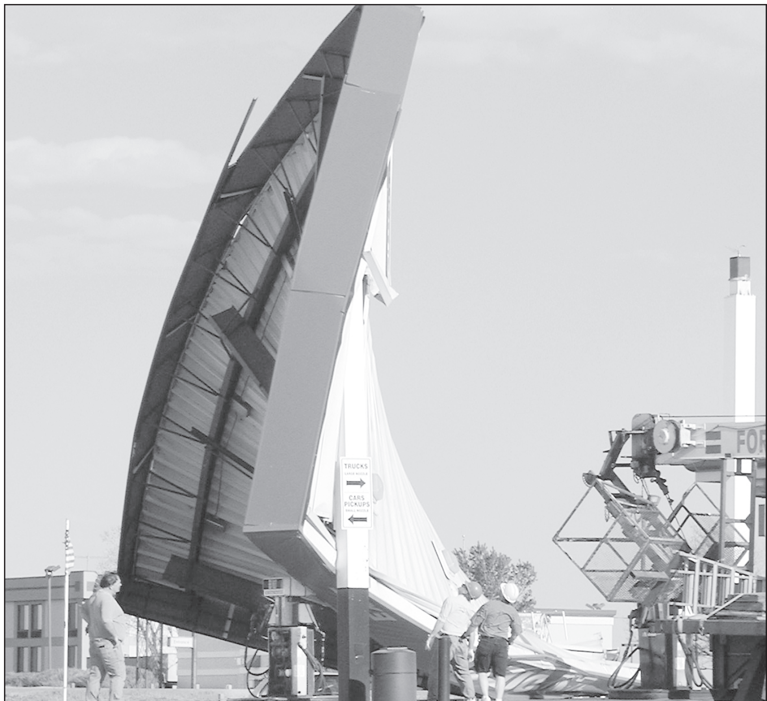
Sustained winds of 50-plus mph took its toll on the canopy at BP 24/7 Saturday. Commercial Sign owner Bruce Bandy and Brad
