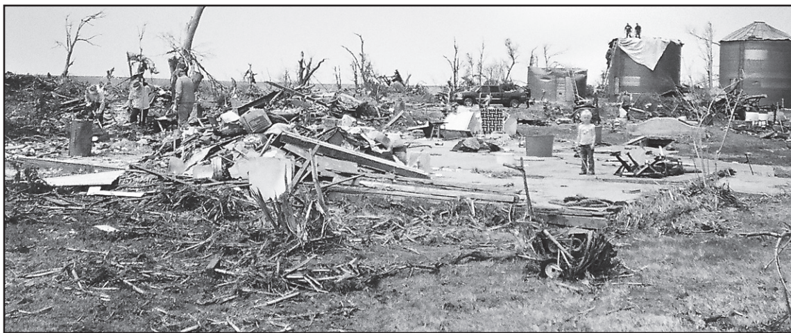
TOP: Residents looked for any shred of their belongings after tornadoes last week in Gove and Sheridan County damaged around 30 homes. LEFT: While some structures remained intact, others had only their foundation remaining as wood and debris covered the ground in parts of both Gove and Sheridan counties.
